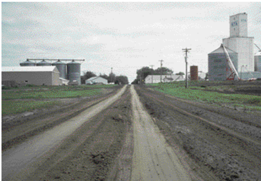
This gravel road shows severe distress after being subjected to a heavy haul from trucks hauling wheat to a grain elevator. The problem was made worse by an unusually wet season.
