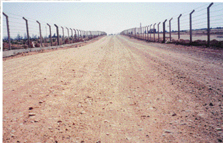
An Egyptian gravel road which is heavily travelled with limited access. Notice that despite the lack of ditches the surface performs well. The reason is that in the arid region of Egypt rainfall averages less than three inches per year. (Courtesy of Ali Selim, SD LTAP, USA)
