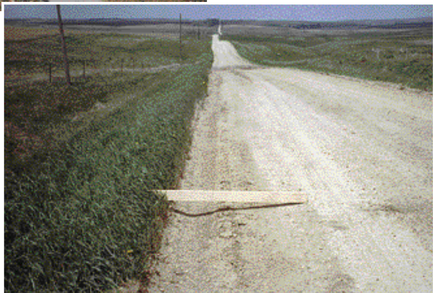
Secondary ditch over six inches deep.
