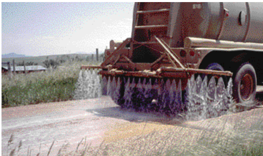
Example of a good piece of application equipment. This truck has a pressurized spray bar with a computerized application system that meters the liquid Chloride with extreme accuracy.
