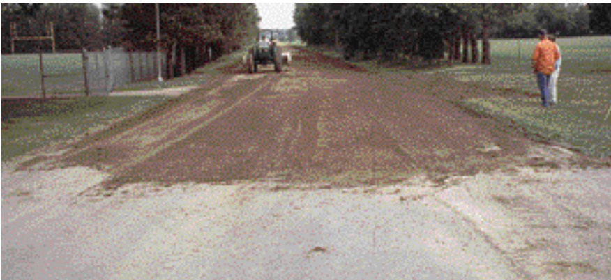
Another washboard-prone area is at the transition from paved to gravel sections as shown in this photo.
